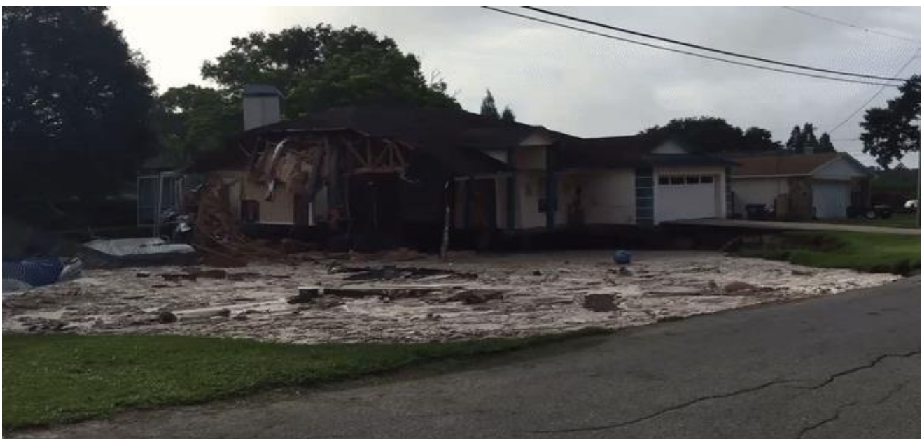
Figure 1.5: Urban/Ground waterflood (Florida 2017)
